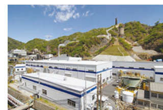
HMC Department, Hitachi Works, JX Metals Smelting
