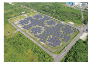
Kudamatsu Mega Solar Power Plant
