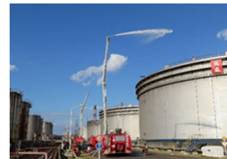
High-altitude chemical water cannon vehicles (Mizushima Refinery)
