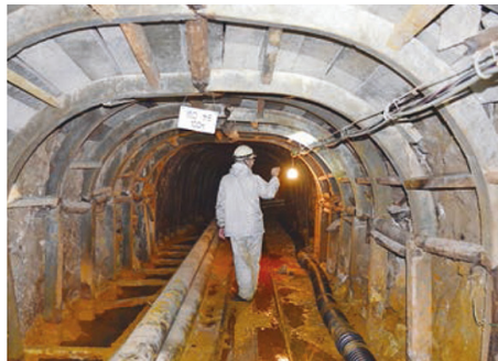
Gallery inspection at Hanawa Mine
