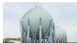
Brace retrofitting on a spherical tank
