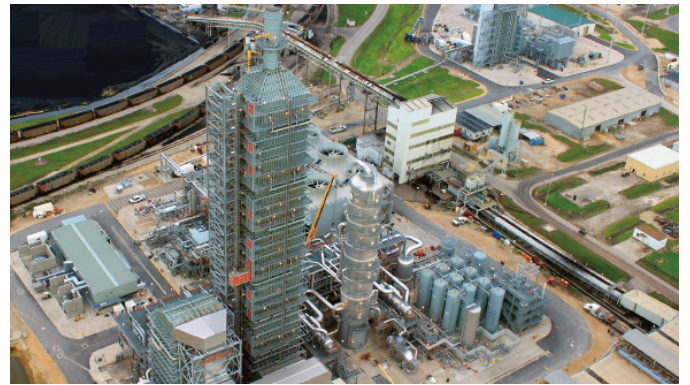
CO 2 recovery plant (state of Texas in the United States)
